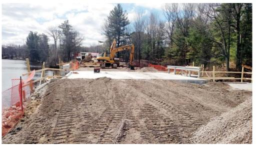
This bridge structure type is the first of its kind to be constructed in the Great Lakes Bay Region and the second in the State of Michigan. The bridge is a GRS-IBS (Geosynthetic Reinforced Soil-Integrated Bridge System) structure that has a 22' span and 7' plus headroom for smaller boat traffic. High strength concrete slabs were used for the bridge deck.
