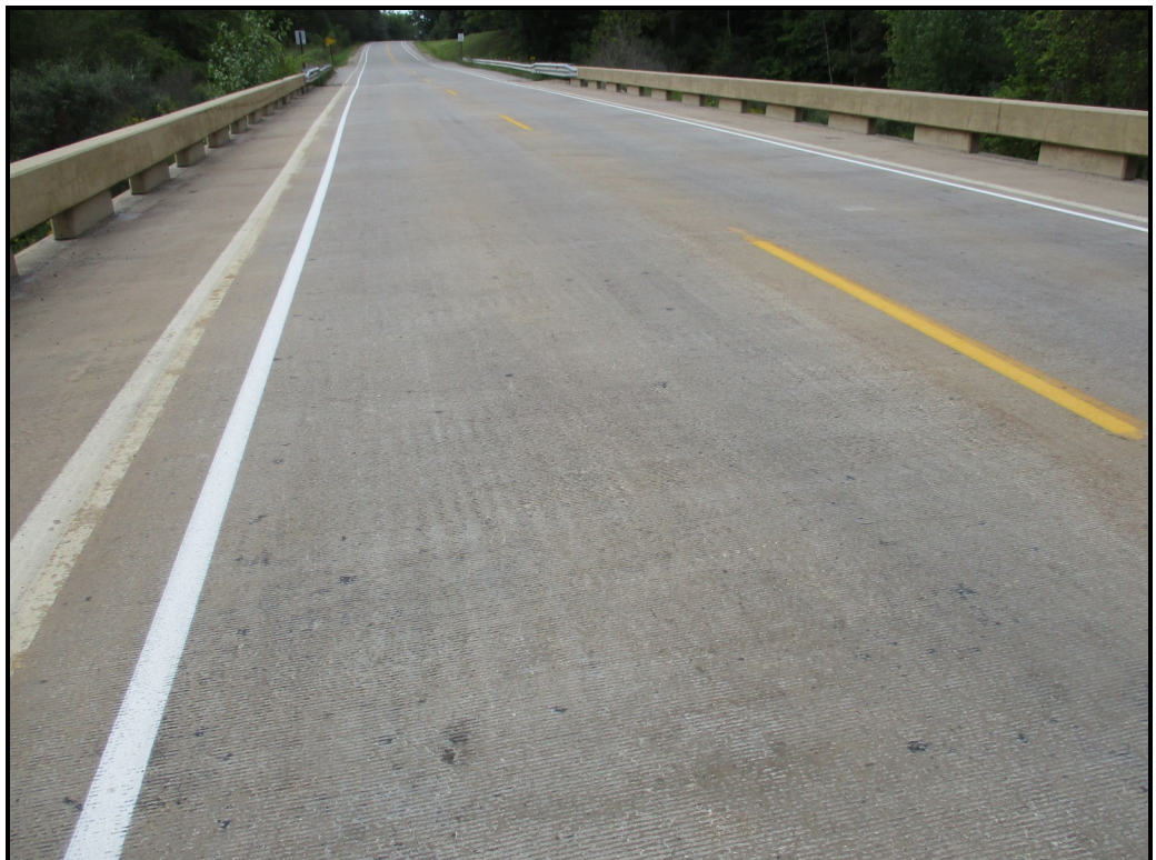
Healer/sealer on concrete deck
