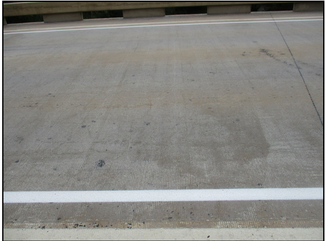
Hairline cracks in surface
