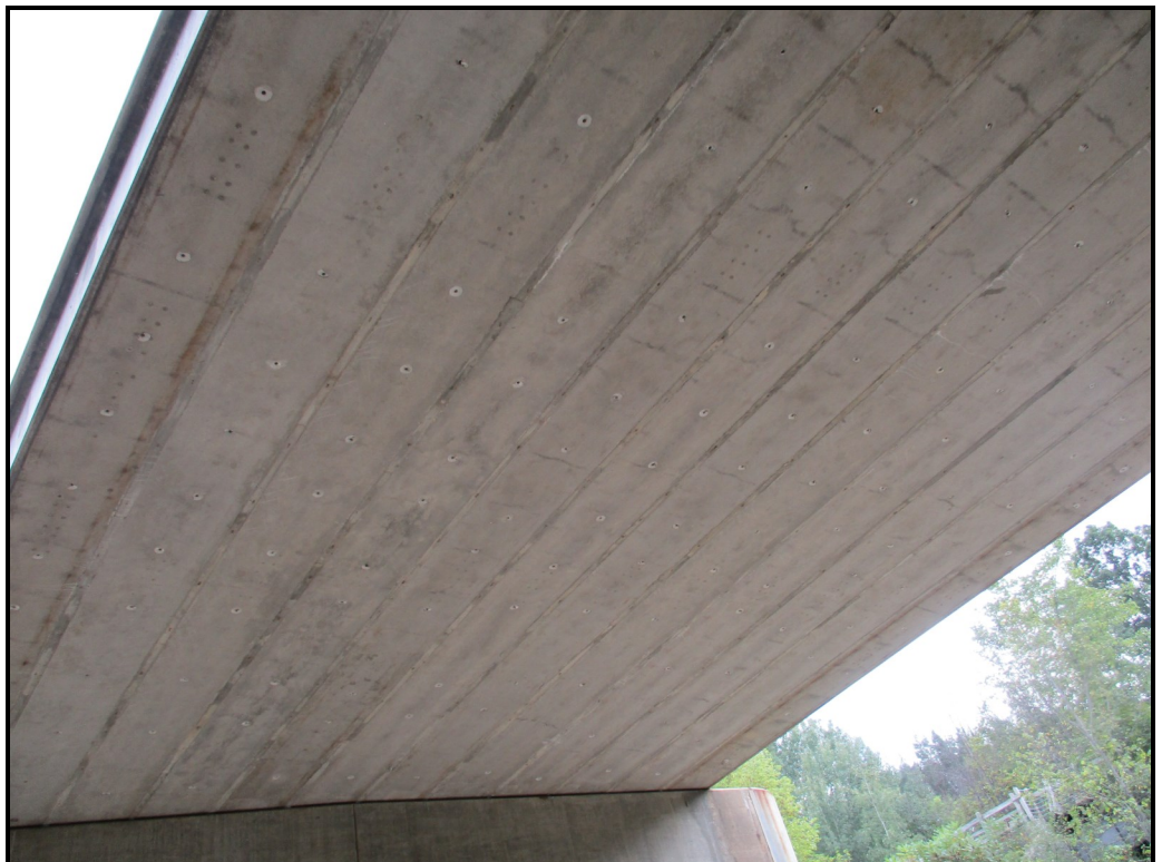
Bottom of box beams
