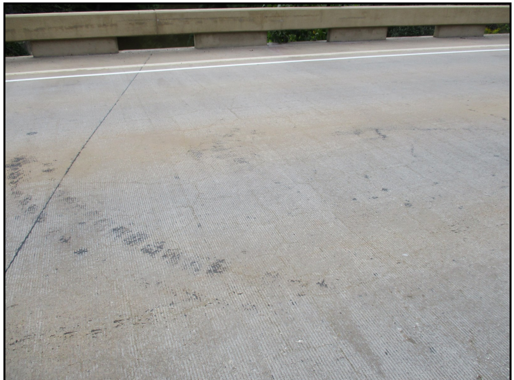
Hairline cracks in surface
