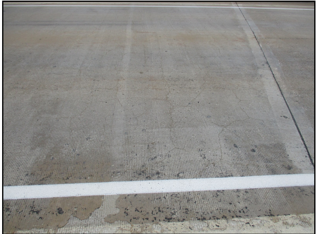
Hairline cracks in surface
