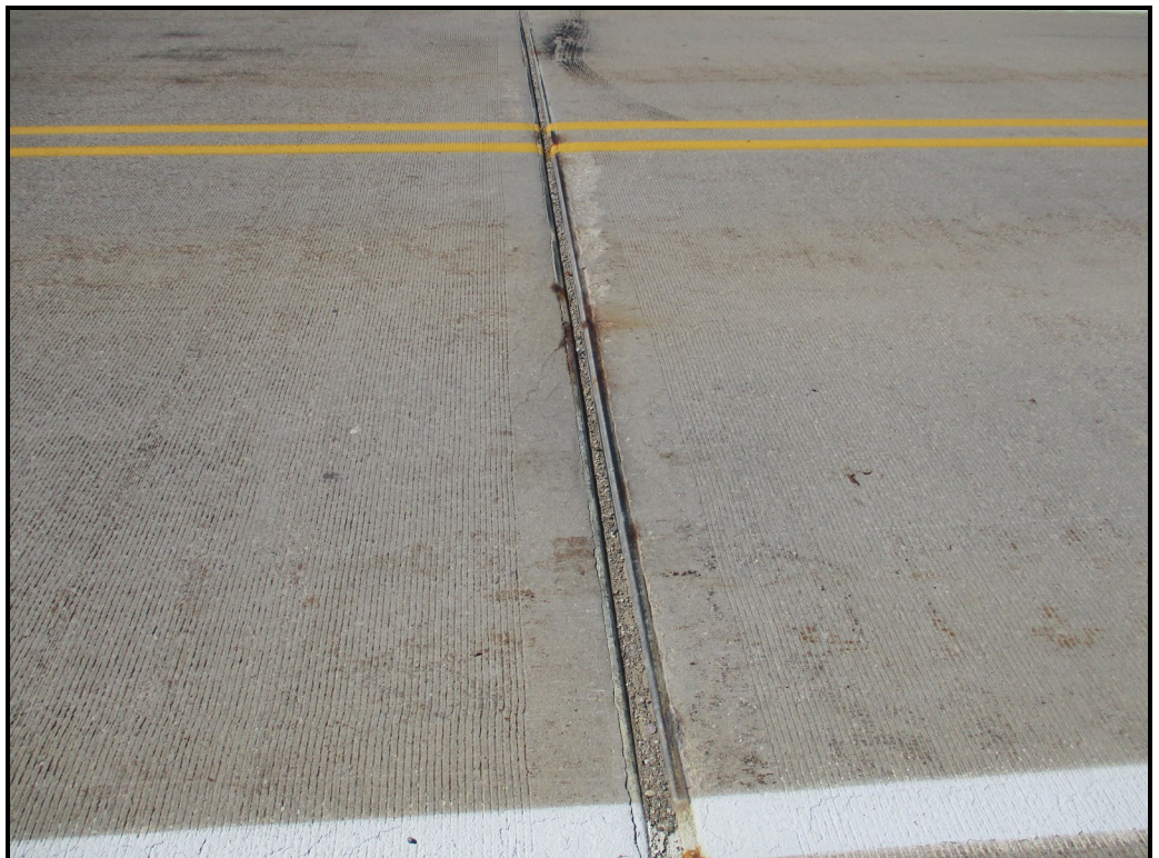
Expansion joint over pier
