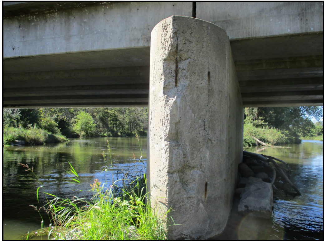
Spalls with exposed steel at east end of pier
