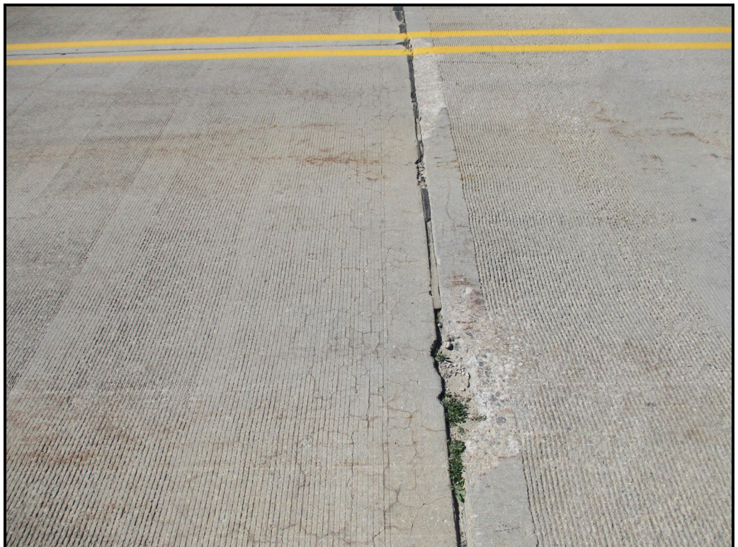
Spalls along south end joint
