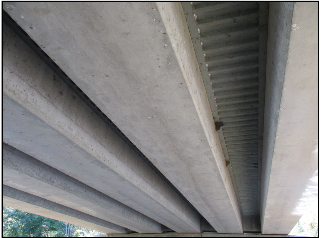
Spread box beams
