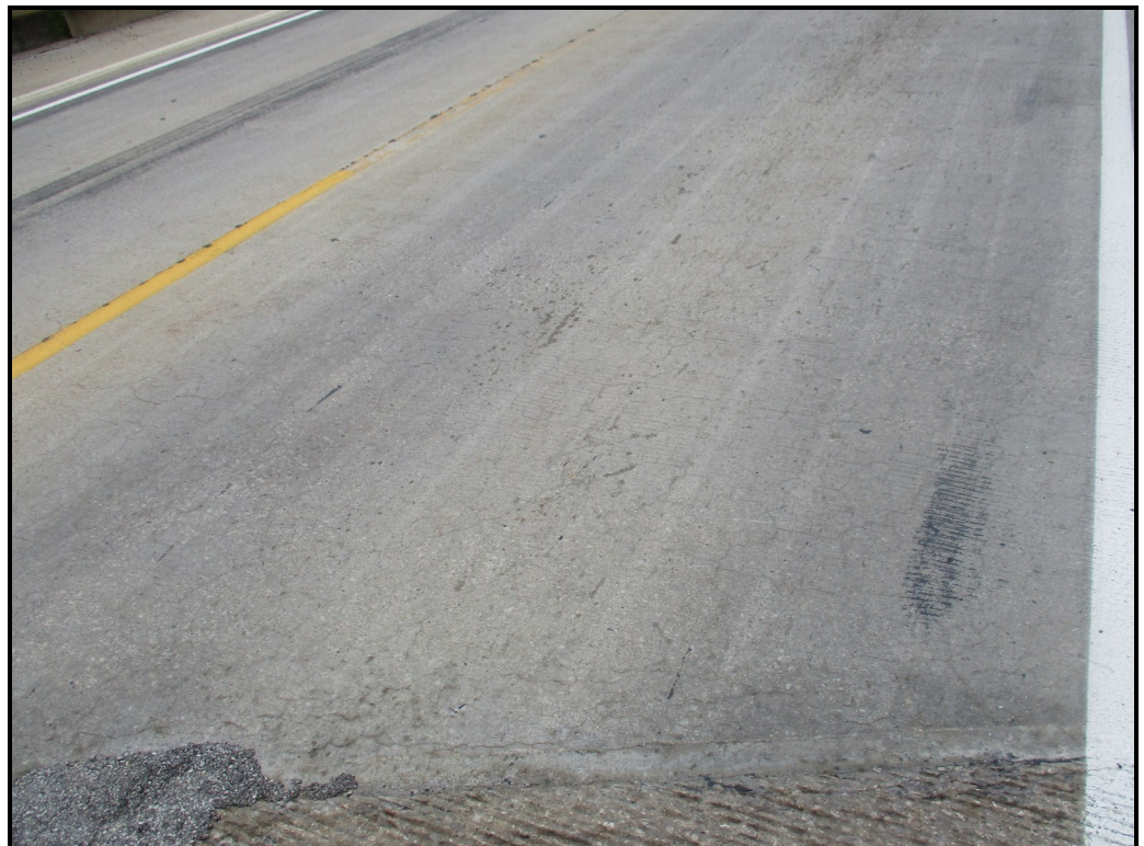
Hairline cracks in surface
