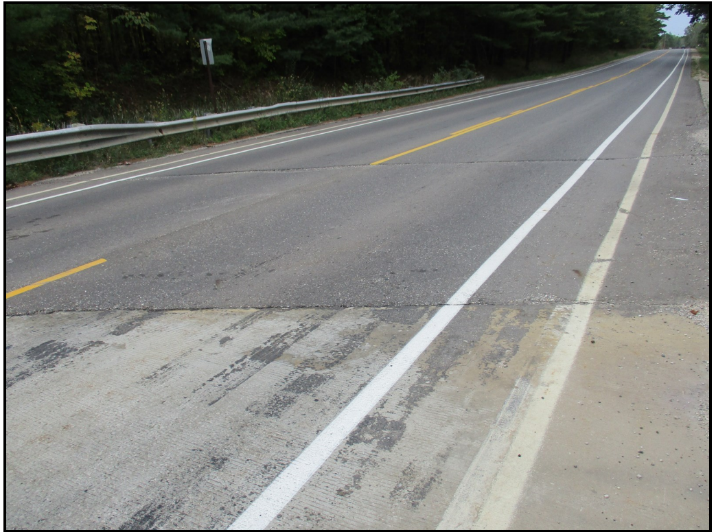
New HMA pavement
