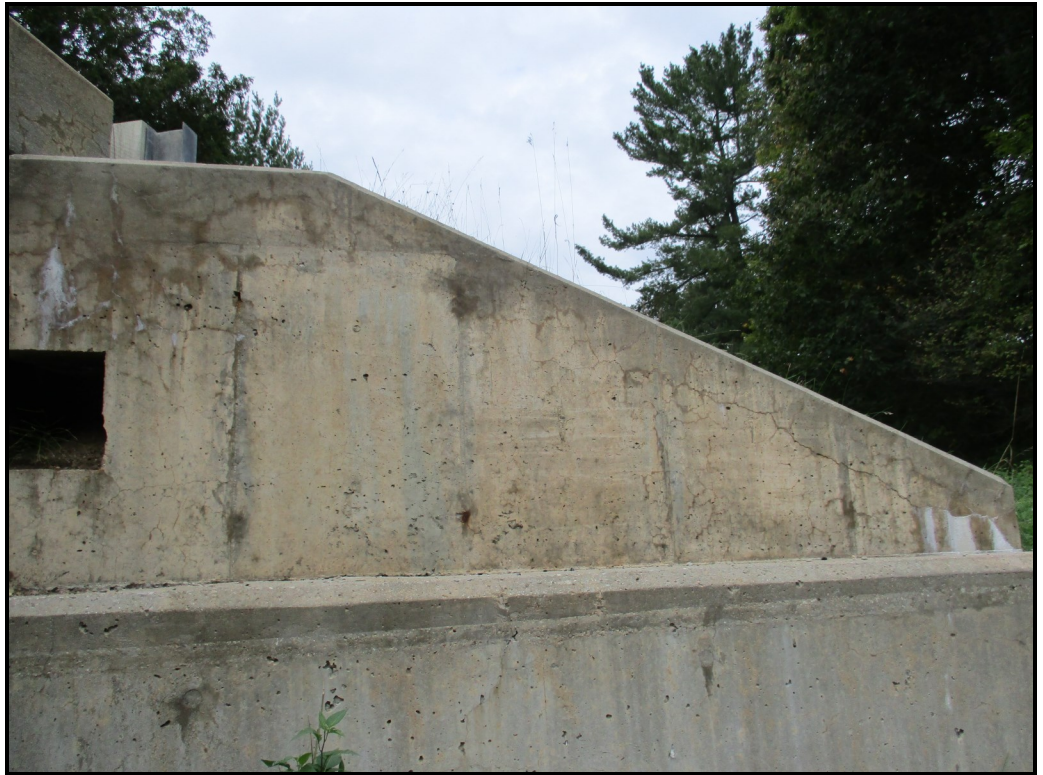
Leaching cracks in slope wall
