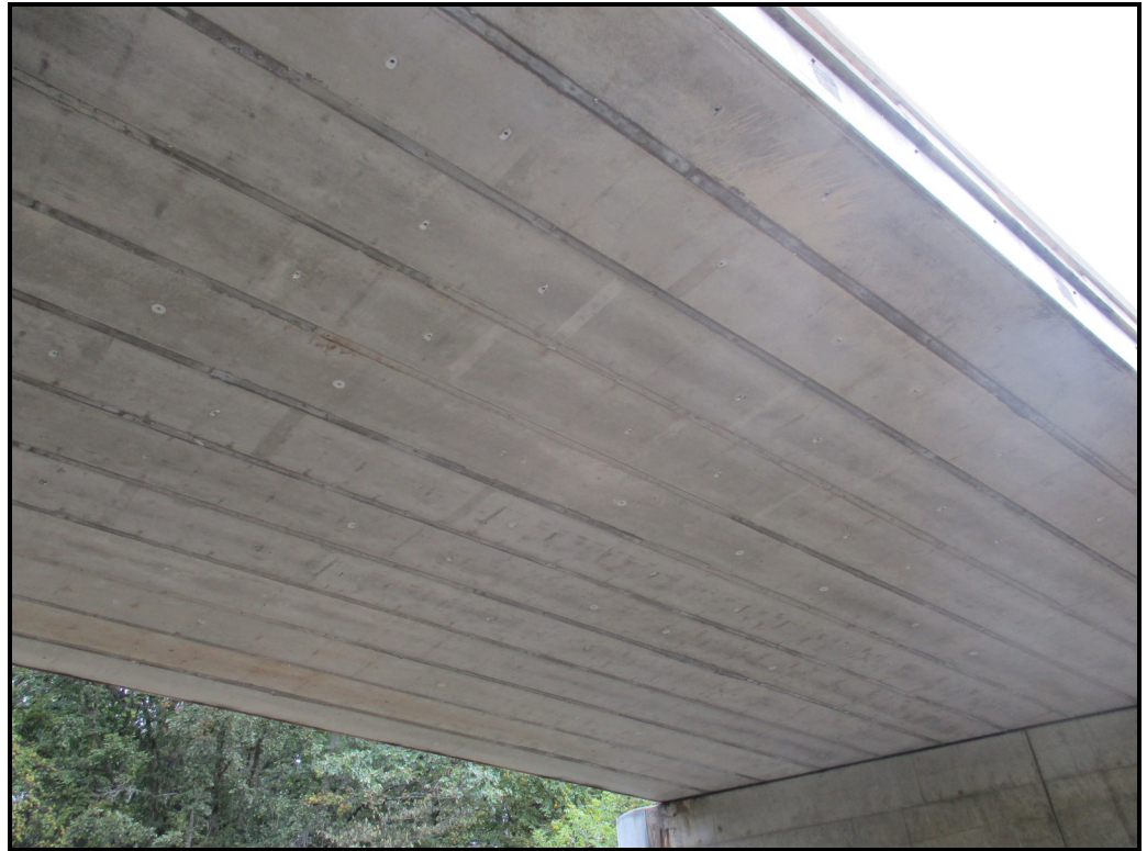
Bottom of box beams
