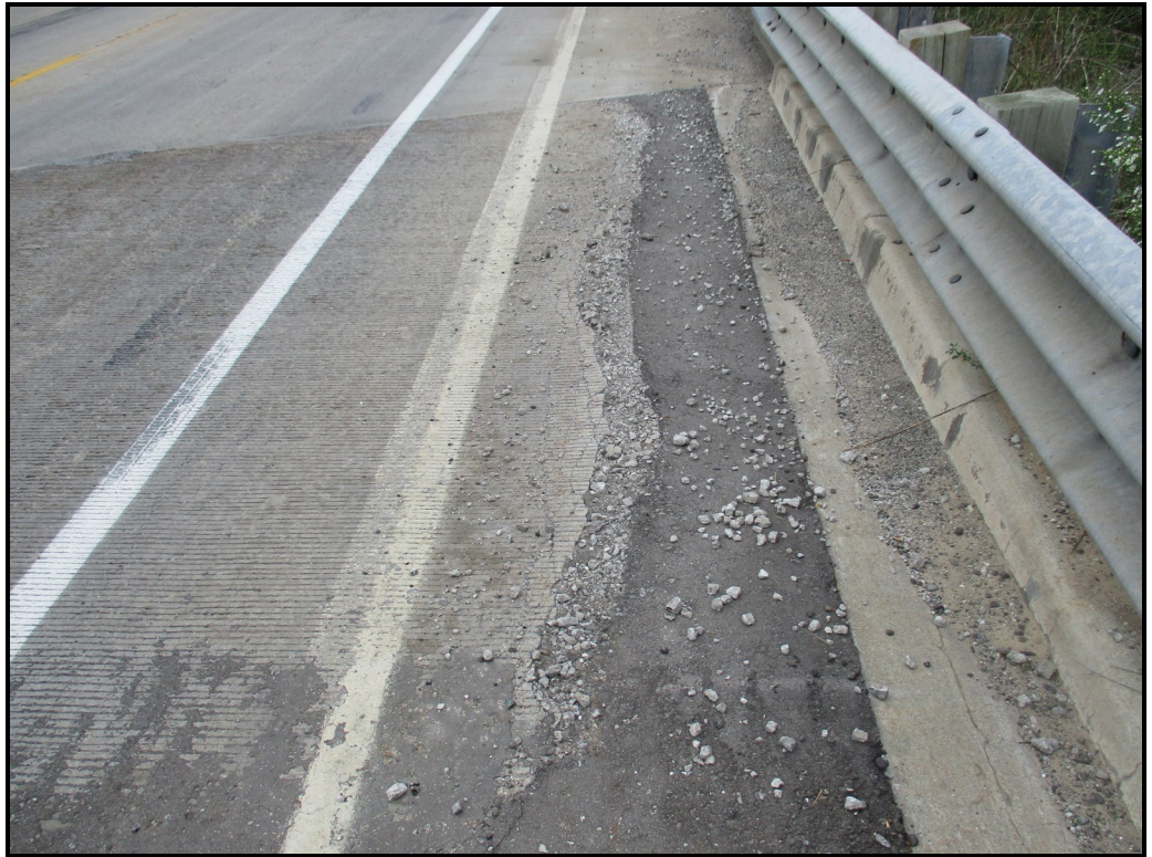
Spalling/HMA patch in approach
