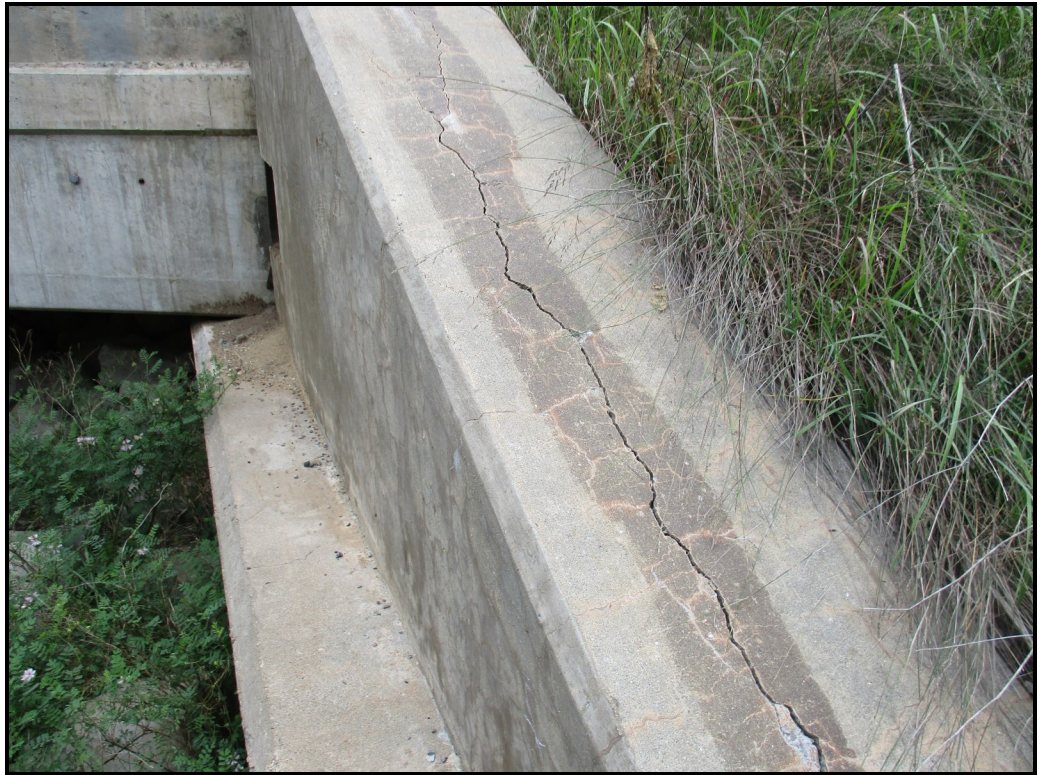
Open crack in slope wall
