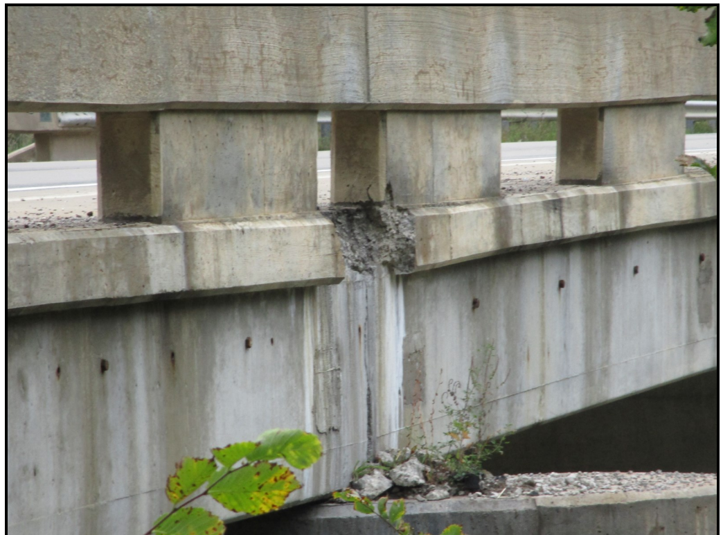
Spall in south deck fascia over west pier
