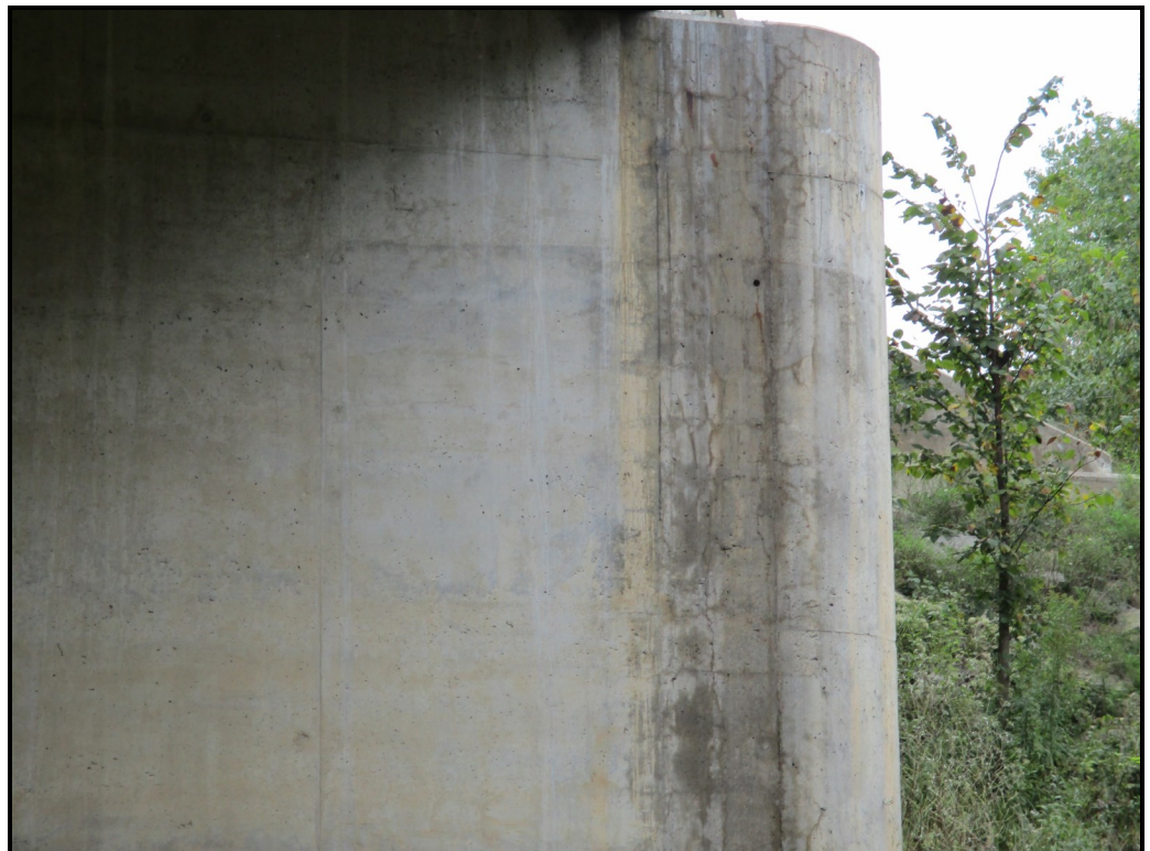
Hairline map cracks at end of pier
