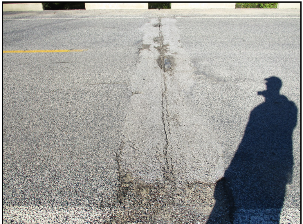
Patching over expansion joint
