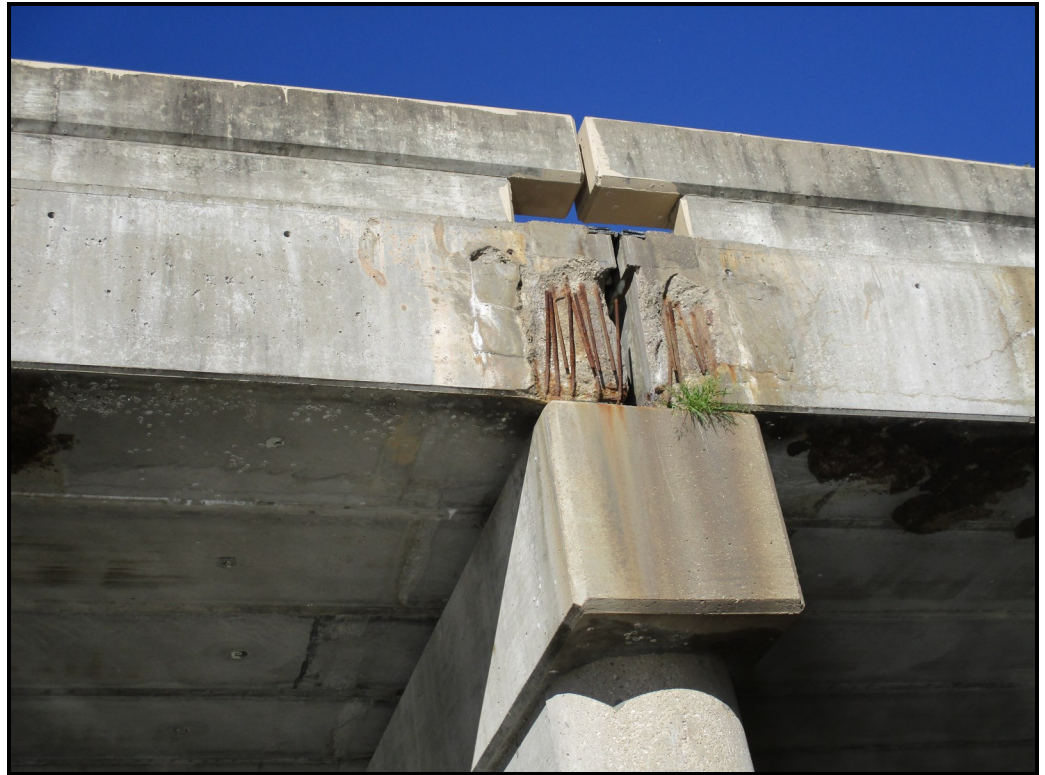
Exposed resteel in east fascia over pier
