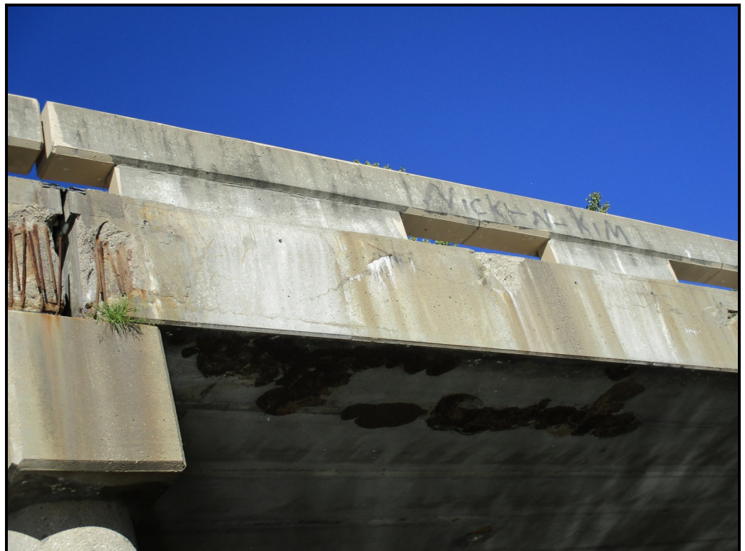
Spall and leaching crack in east fascia, north span
