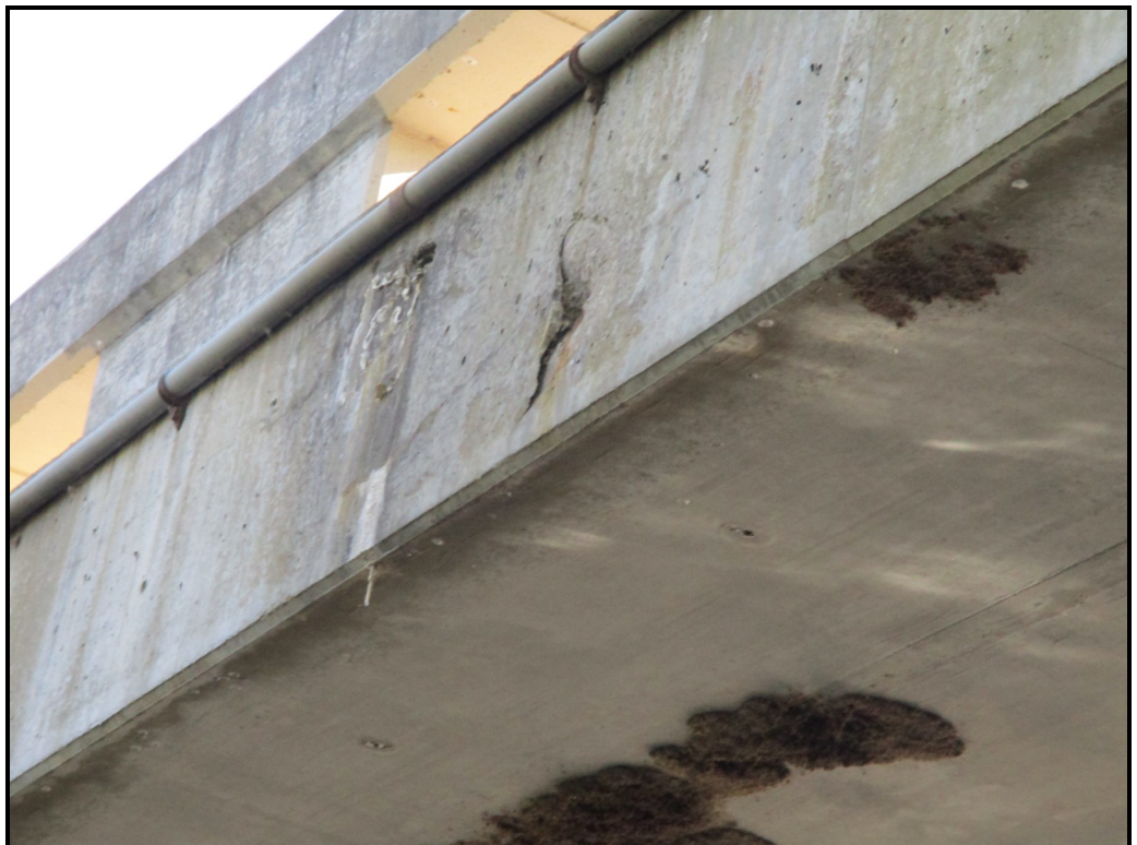
Spall in west fascia, south span
