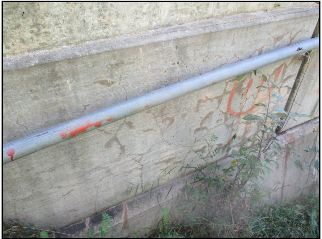
ASR cracks in north abutment
