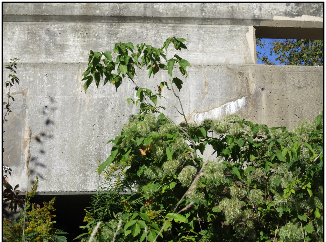
Leaching shear crack in east fascia beam
