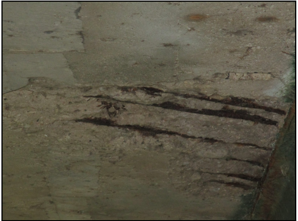
Spall with exposed steel in deck bottom
