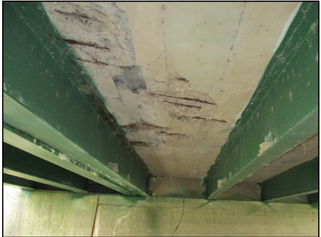
Spalls in deck bottom
