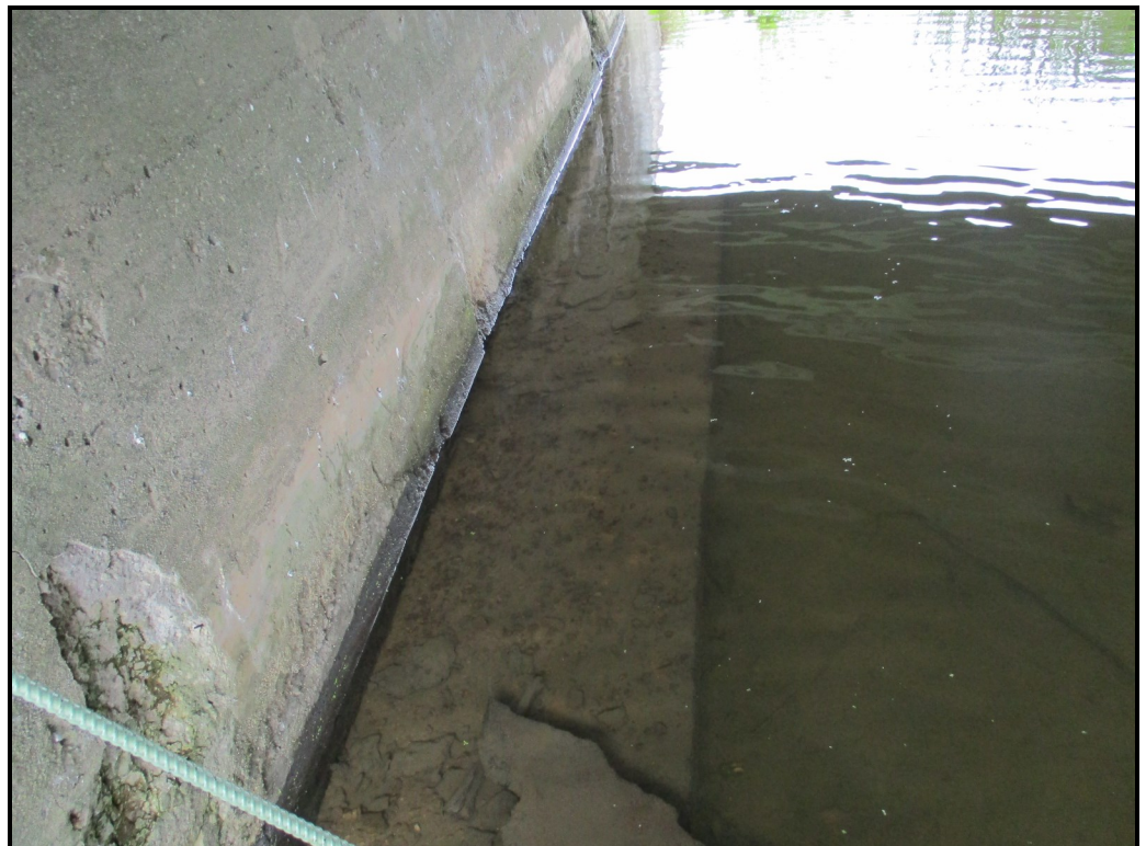
Exposed footing, typical
