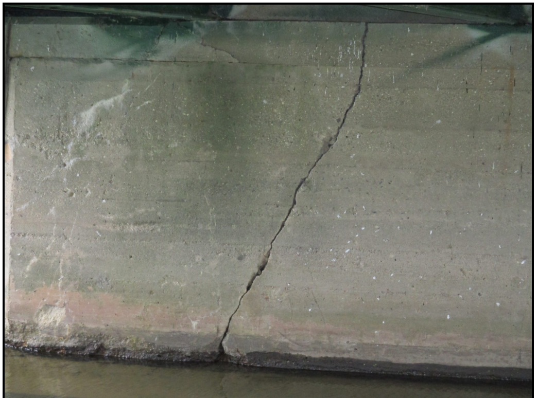
Vertical crack in east abutment
