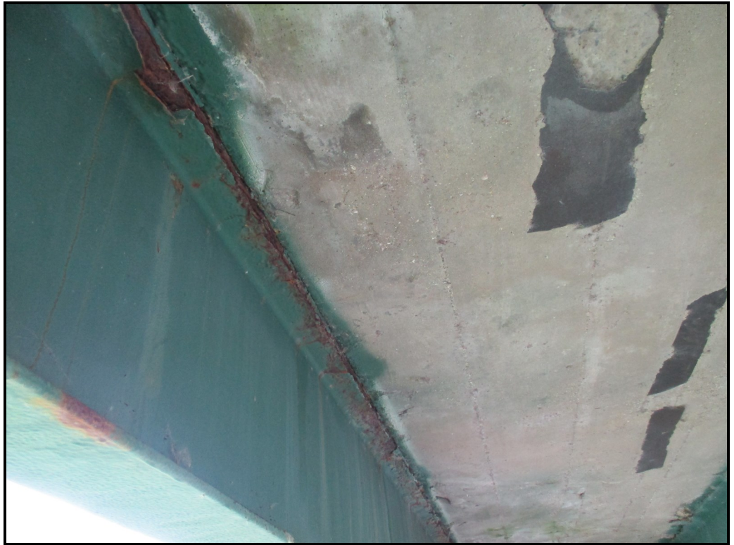
Rust and scale along top flange
