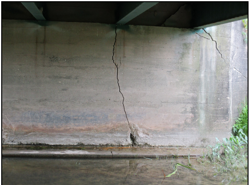
Crack in south abutment
