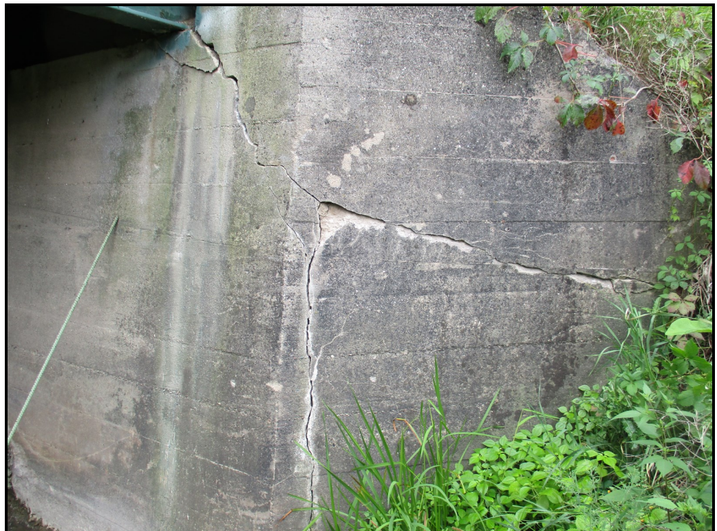
Crack in SW wingwall
