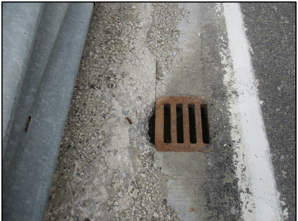
Spalled brush block face at deck drain
