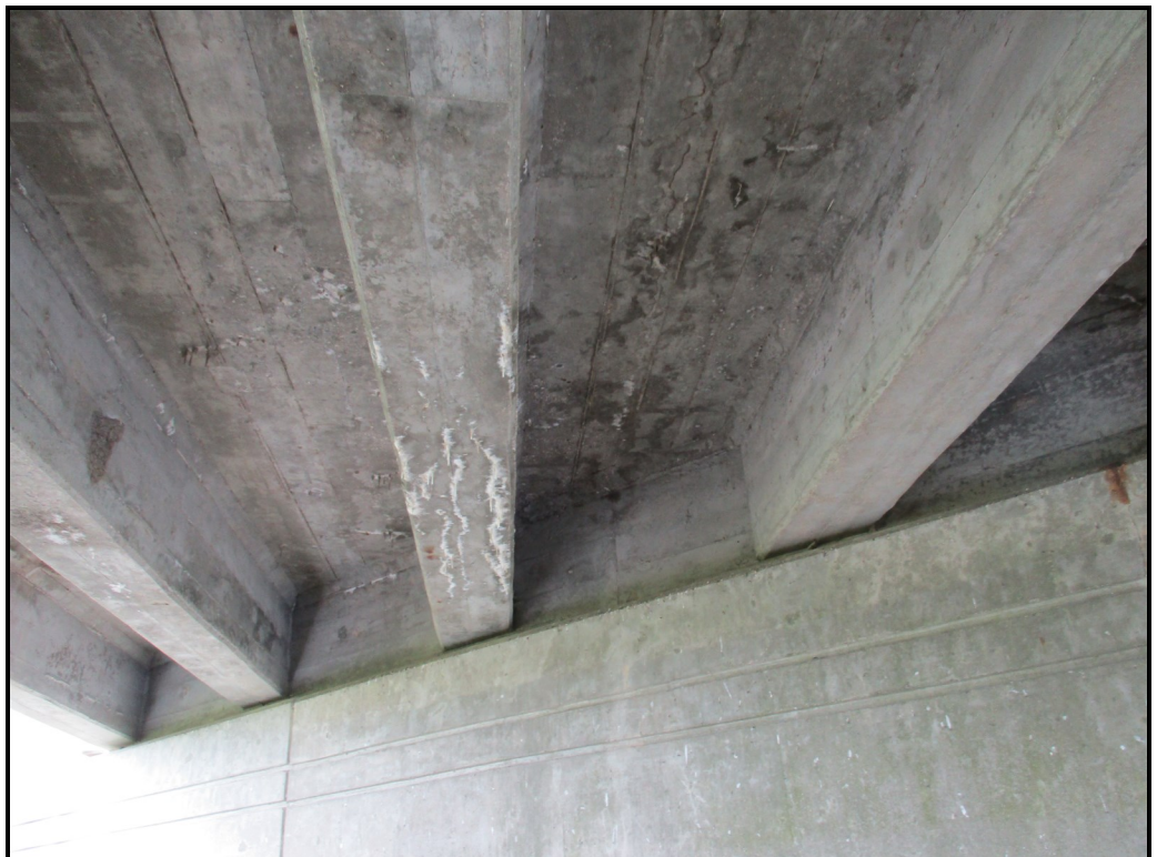
Leaching cracks in bottom of tee beam
