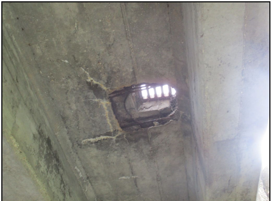
Spall in deck bottom with exposed steel
