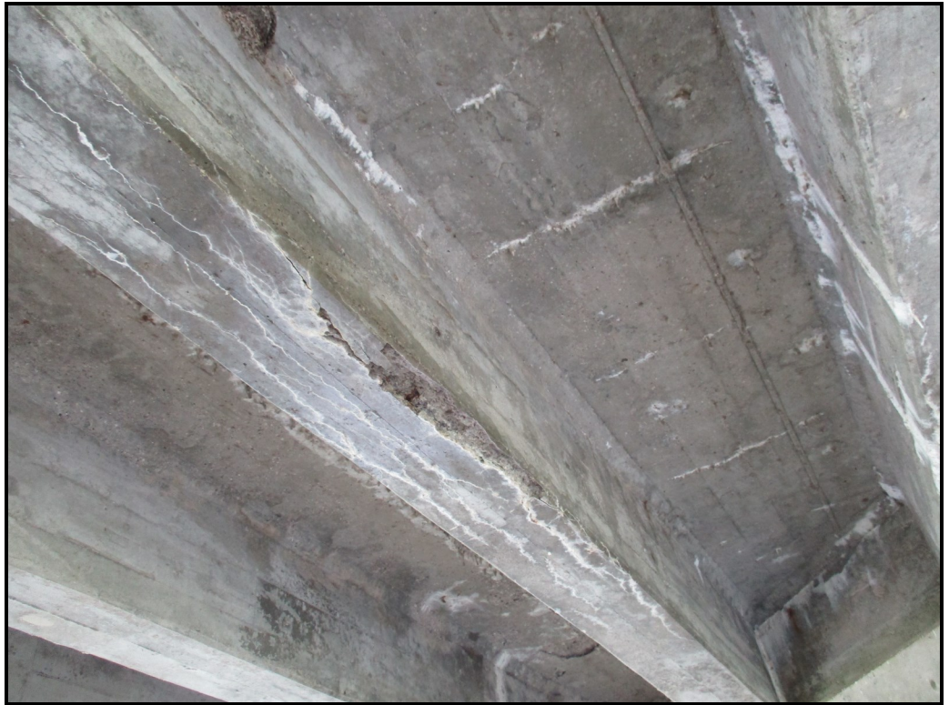
Spall with exposed steel in beam 3W
