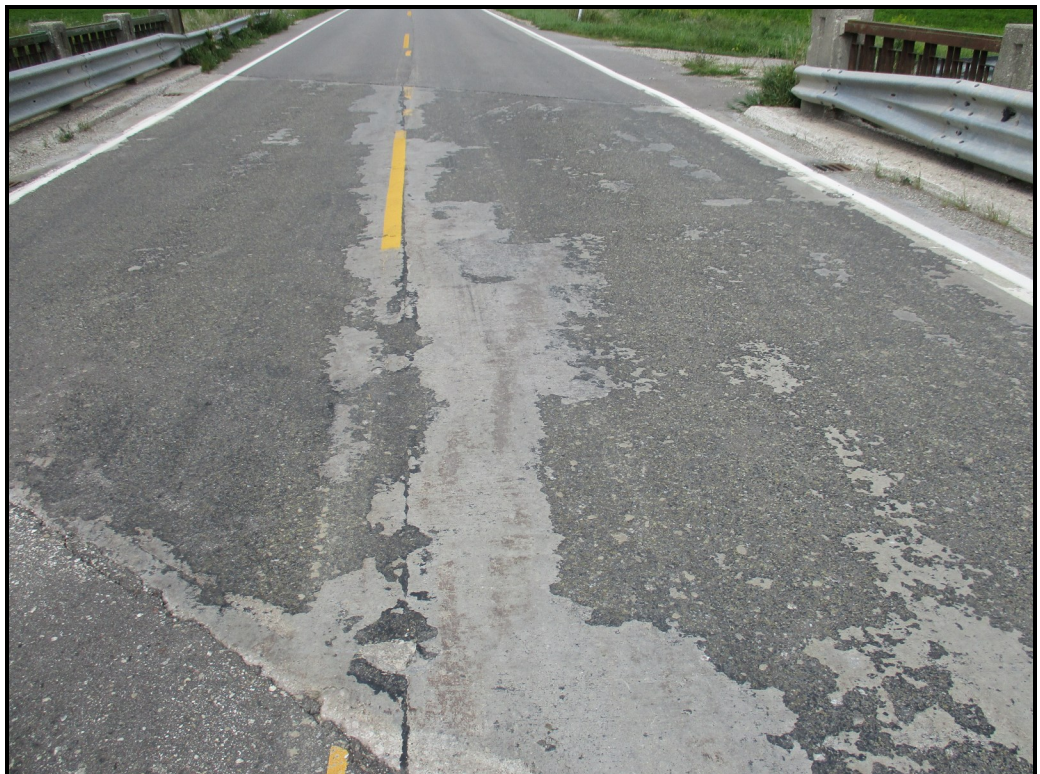
Chip seal peeling off of concrete surface
