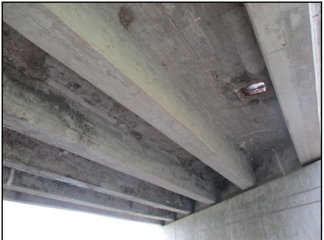
Concrete tee beams
